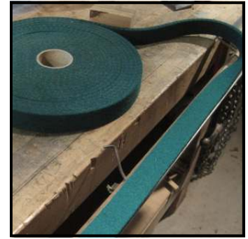
New cloth being installed
