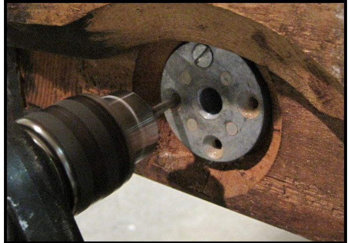
New socket being installed.
